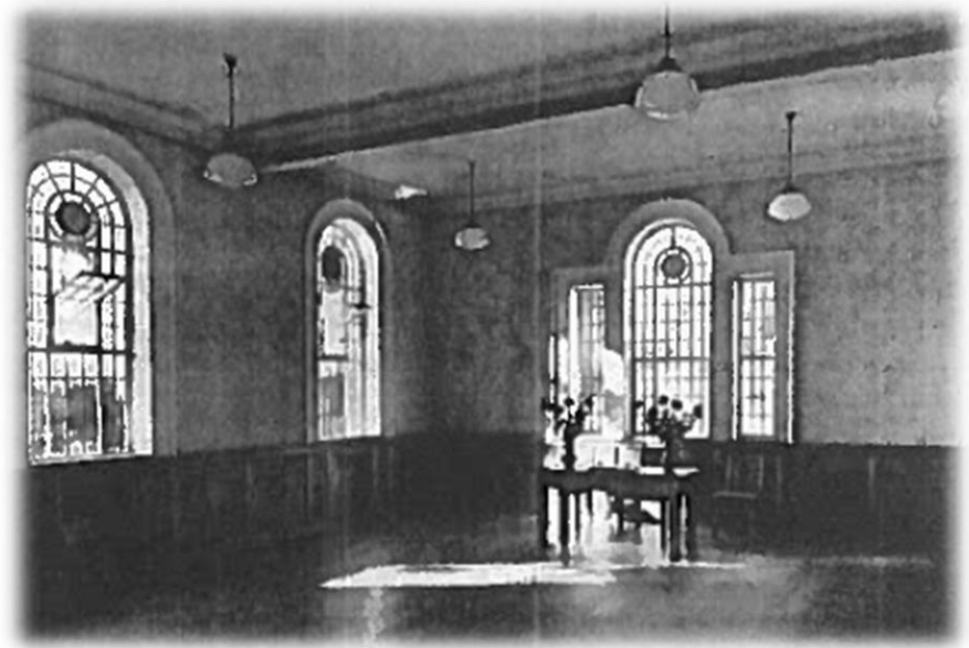
Figure 4 - Interior of the Memorial Hall (Photo by Cosser Photographic Service)
